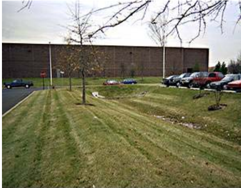
Grassed swales can be used along roadsides and parking lots to collect and treat storm water runoff
